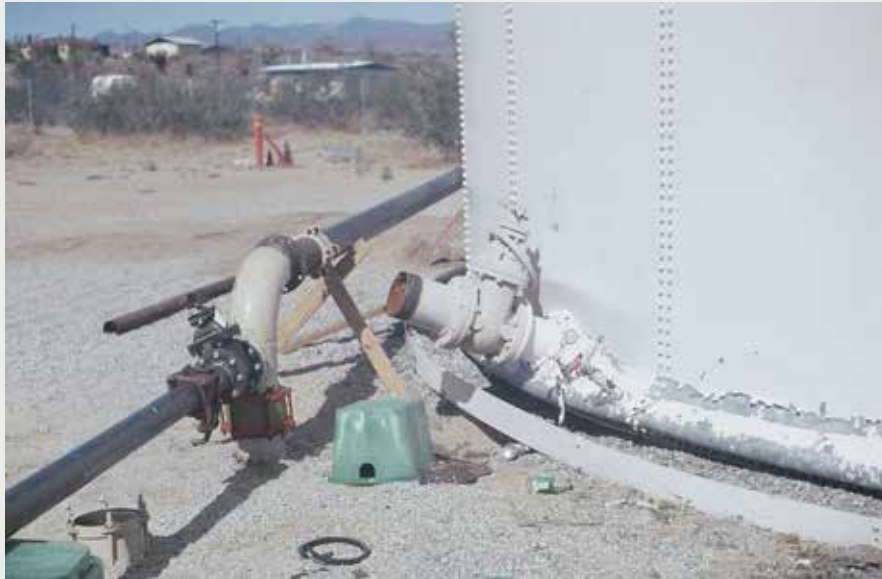
Water sloshing lifted this tank off the ground causing pipeline separation and elephant foot failure during 1992 Landers earthquake in San Diego.
