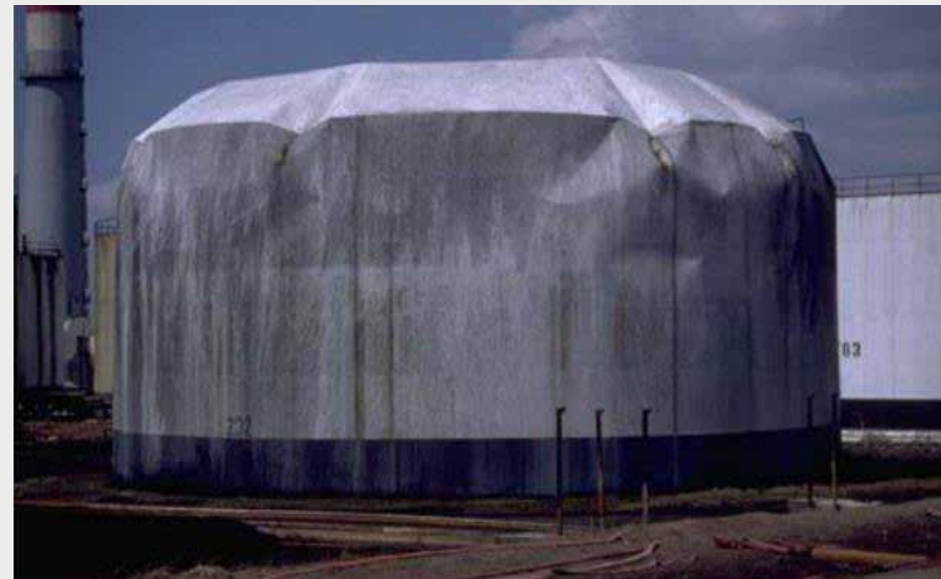
Sloshing damage to upper shell and roof of tank during 1999 earthquake in Turkey
