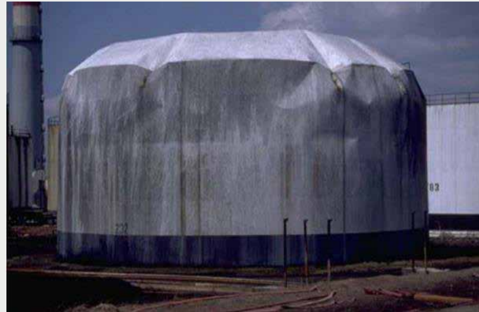
Sloshing damage to upper shell and roof of tank during 1999 earthquake in Turkey
