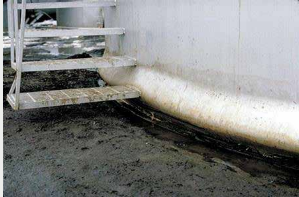
Elephant's foot buckle at the base of a storage tank during 1964 earthquake in Alaska
