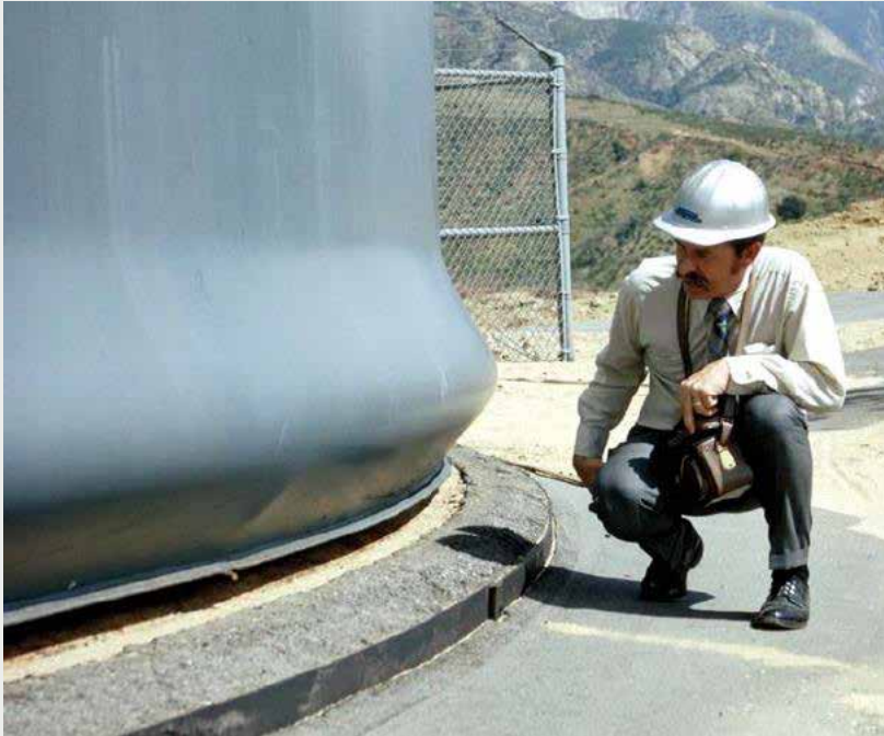
Fluid-filled tank buckled in "elephant-foot" mode during Northridge earthquake in California
