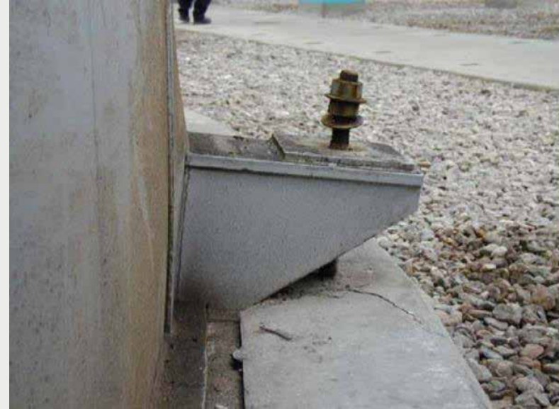
Lengthening the anchor rod, deformation of tank (5000 m 3 oil), and concrete cracking during 2001 earthquake in Peru
