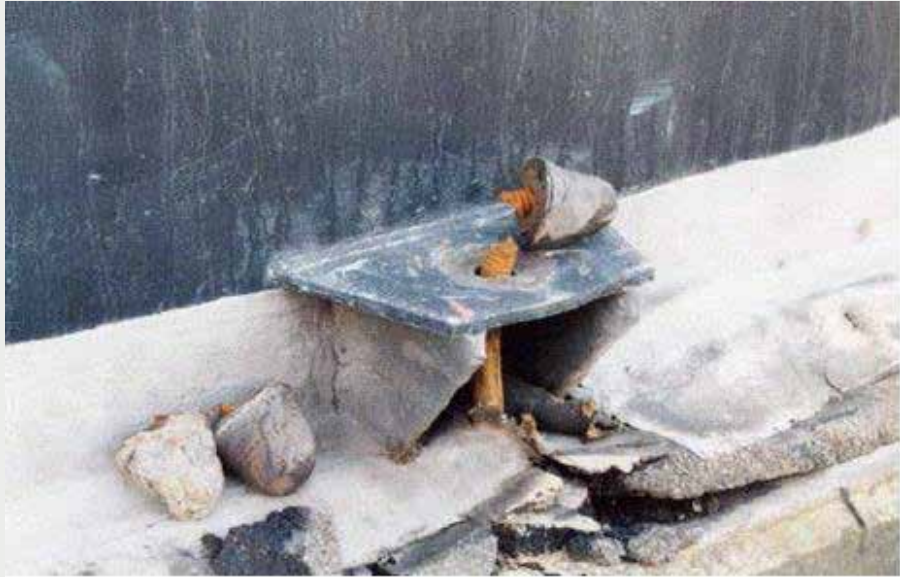
Fracture of tank anchors during 1995 earthquake in Japan
