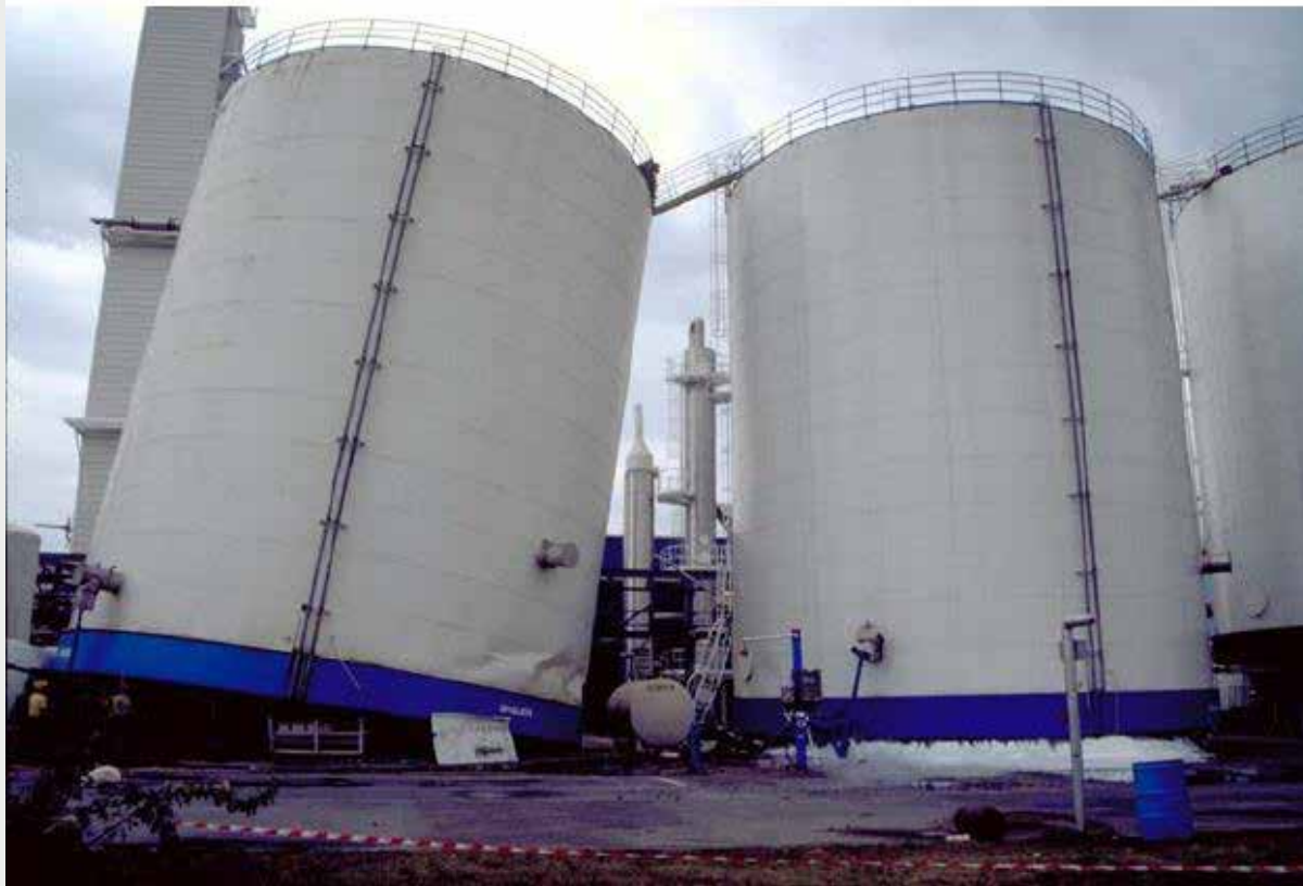
Failure of concrete piles supporting Liquid oxygen tanks during the 1999 Izmit earthquake in Turkey
