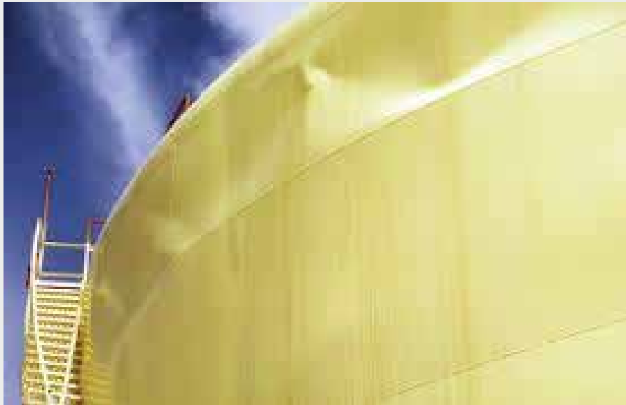
Sloshing damage to upper shell of tank during 1971 earthquake in California
