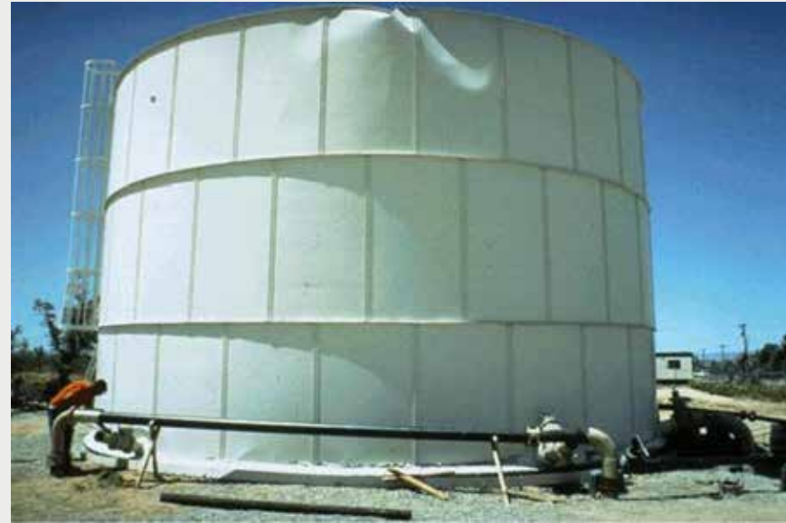
Damage at the top of the tank where water in the tank pushed up on the roof during 1992 Landers earthquake in San Diego
