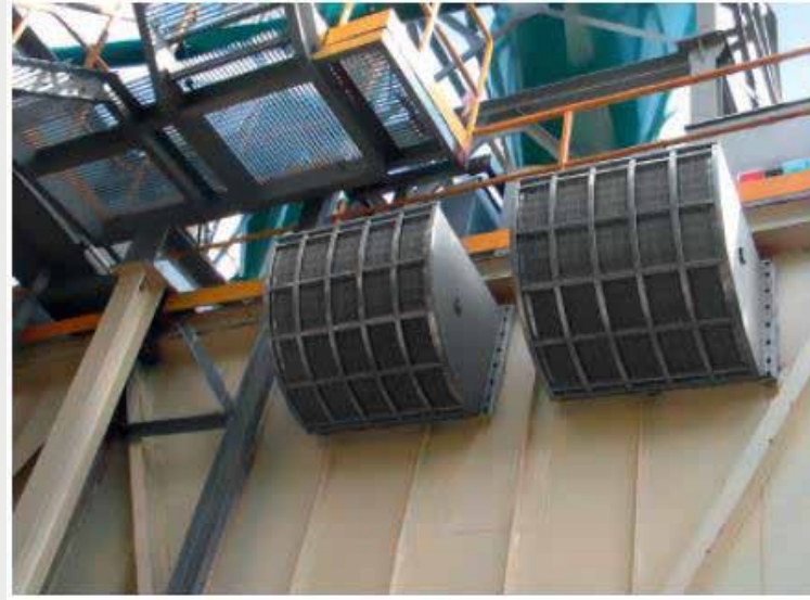
Explosion venting of a chip bunker using the Q-Box to protect the surrounding infrastructure.
