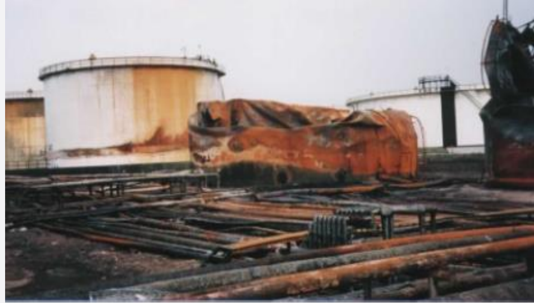
Collapsed tanks and piping system in tank farm due to fire after the Kocaeli Earthquake in Turkey in 1999
