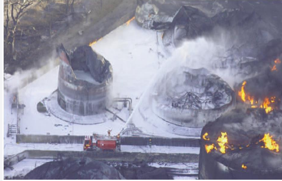
Response of a partially filled tank to blast within the shallow cloud (Buncefield explosion)
